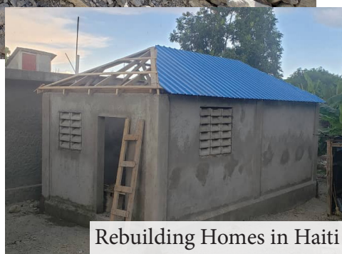
Rebuilding Homes in Haiti
